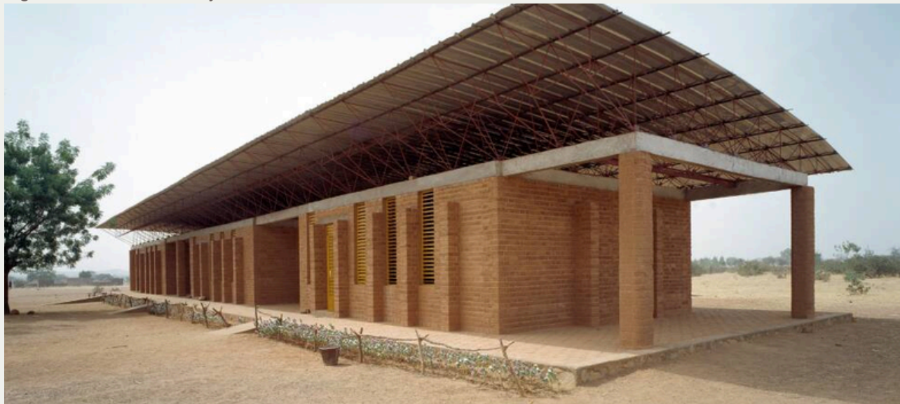
Figura 11. Gando Primary School
