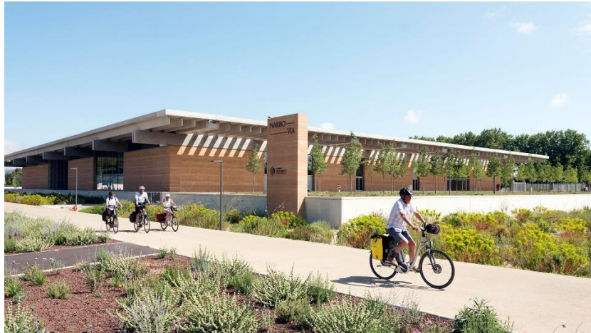
Ilustración 5: Foster and Partners. (s.f). Narbo Via [Fotografía]. En Foster + Partners. Recuperado de https://www.fosterandpartners.com/projects/narbo-via
